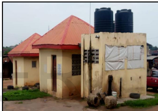
Figure 7. Sample of Water Flush Public Toilet at Owode Lagos Garage
